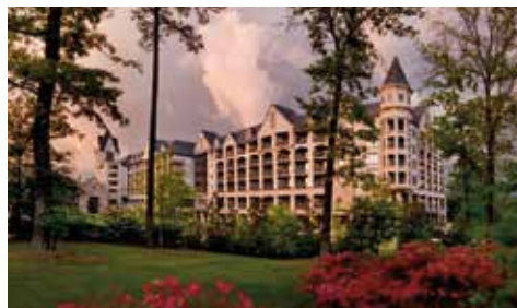
Renaissance Birmingham Ross Bridge Golf Resort & Spa
