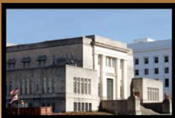
OLD JUDICIAL BUILDING RENOVATION & OFFICE COMPLEX- MONTGOMERY under construction / Completion Date: 2010 © TIM L. PHILLIPS, CCP
