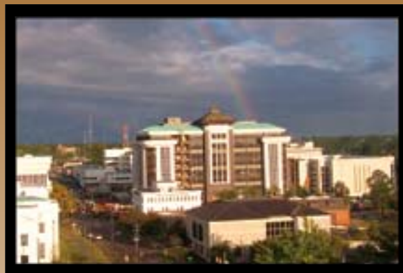
THE RETIREMENT SYSTEMS OF ALABAMA HEADQUARTERS BUILDING- MONTGOMERY under construction / Completion Date: Summer 2008 © TIM L. PHILLIPS, CCP
