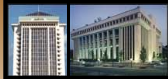
RSA TOWER / RSA PLAZA, Montgomery
