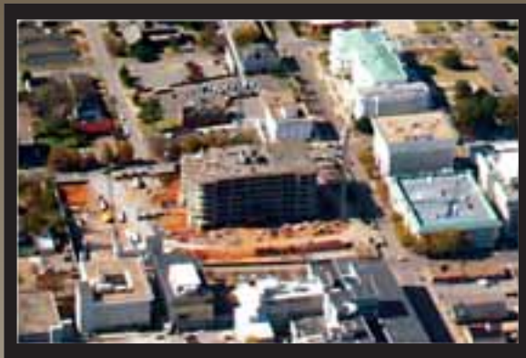
THE RETIREMENT SYSTEMS OF ALABAMA ADMINISTRATION BUILDING - MONTGOMERY under construction / Completion Date: Early 2008
