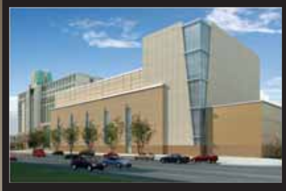
THE PERFORMING ARTS CENTER - MONTGOMERY Completion Date: Early 2008
