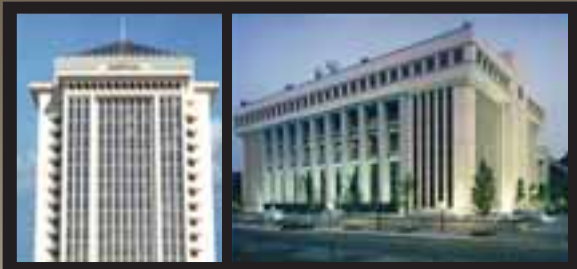
RSA TOWER / RSA PLAZA, Montgomery
